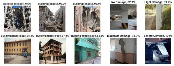
Figure 4. AI-based evaluation of structural damage state (a) system level; (b) component level
