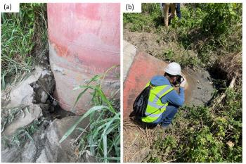
Figure 4. Signs of soil liquefaction around pier foundations of (a) New Xiuguluan River Bridge pier #12 (view from the east side) (b) Gaoliao Bridge that is tipping-over
