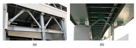
Figure 1. The installation of hysteretic dampers: (a) in buildings, (b) under bridges
