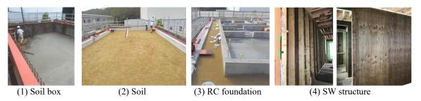
Figure 4. B-building with Foundation-soil system (Upper structure: SW structure)
