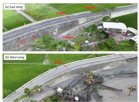
Figure 5. Overview of ramp embankments at east and west wings of Gaoliao Bridge
