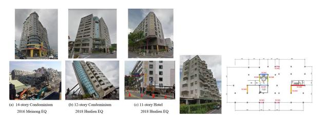
Fig. 3- Collapsed buildings with soft first story
