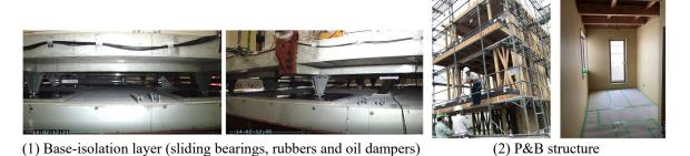
Figure 3. A-building with Base-isolation system (Upper structure: P&B structure)
