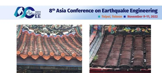
Figure 5. Conventional roofing tiles of masonry temples. Left: Tongban, convex tile; Right: Yanho, red tile.
