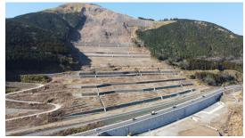
(a) Slope stability works for Tateno landslide
