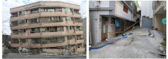
(a)Structural damage (b)Building settlement by soil liquefaction Figure 1. The damage model of buildings in 20160206 Meinong earthquake
