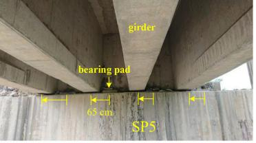
Fig. 13 Large permanent girder displacement at SP5
