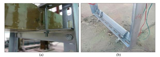
Figure 12. (a) Deformation of the ground braced frame; (b) Failure of the anchor bolt
