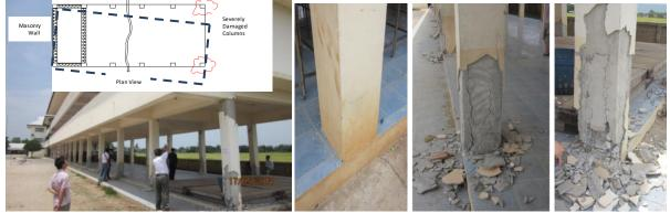
Figure 2. School building damaged by soft story and torsional irregularity.
