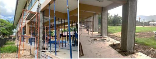
Figure 7. Column Jacketing during construction.
