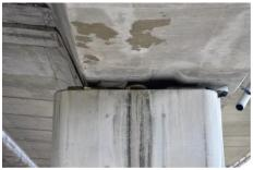
(a) Excessive lateral displacement of girder
