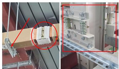
Figure 1. Physical joint and fixing of busway
