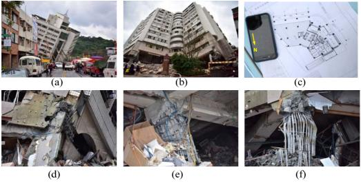
Figure 6. (a) Front view, (b) back view, (c) drawing of floor plan, (d) corner column, and (e) and (f) bottom columns of the collapsed 12-story mixed-use apartment block.
