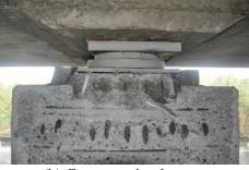
(b) Concrete pier damage
