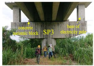
Fig. 12 No permanent girder displacement at SP3
