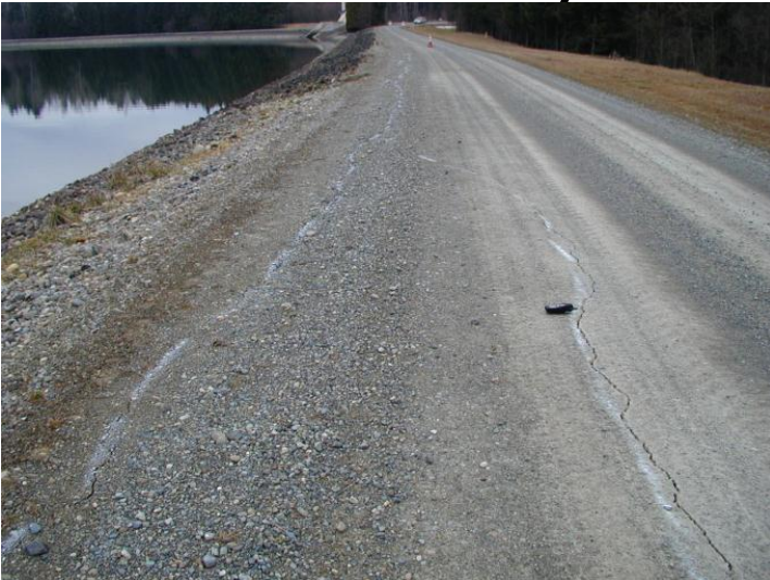
Minor Crack Dam Crack
