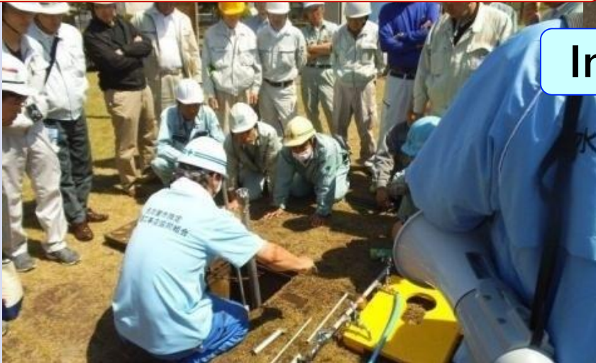
Installing temporary water faucet
