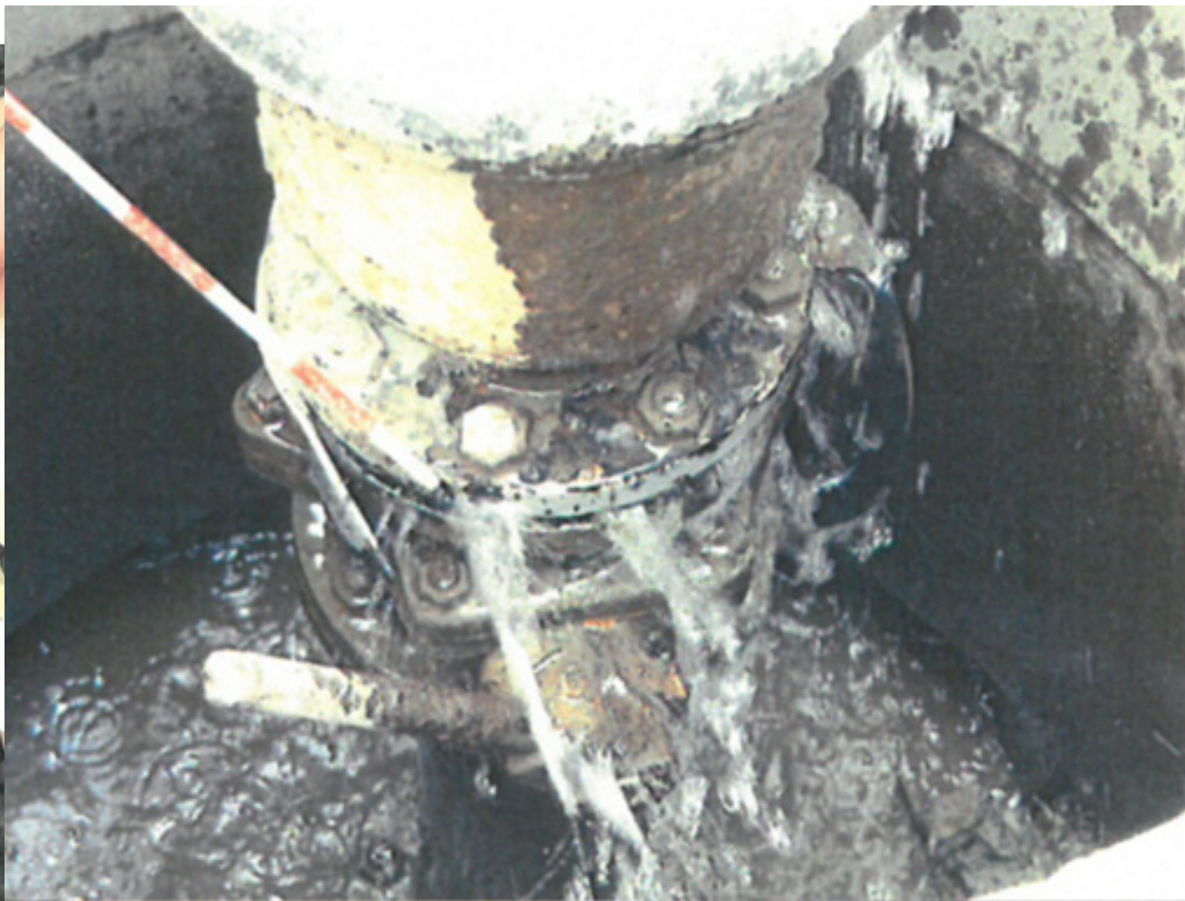
Leakage from flange joint
