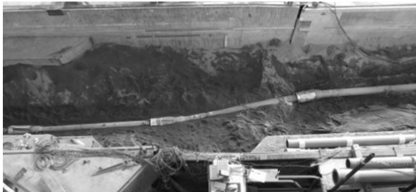
Figure 11. Test specimen after the test
