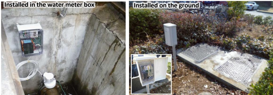
**Photo 5 Installed Data Conversion/Transmission Apparatus**
