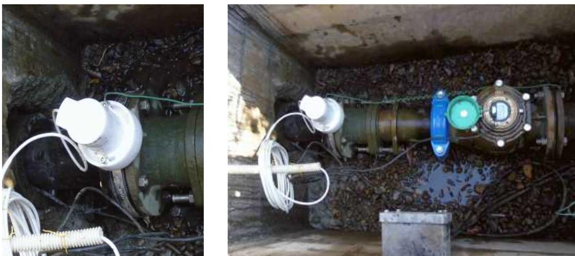
Photo 4 Installation of Pressure Sensor
