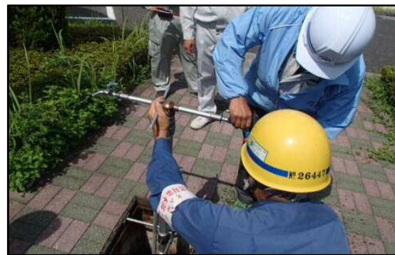
(b) Training on installing temporary water faucets
