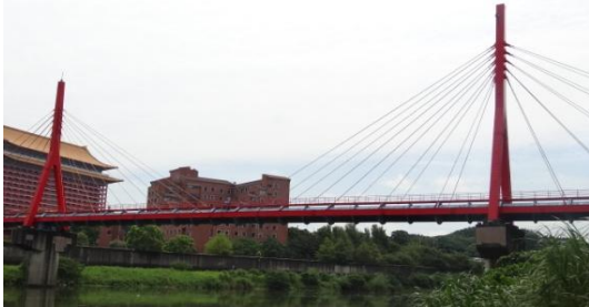
Jiantan cable-stayed water pipe bridge
