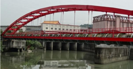
Yuanshan arch water pipe bridge
