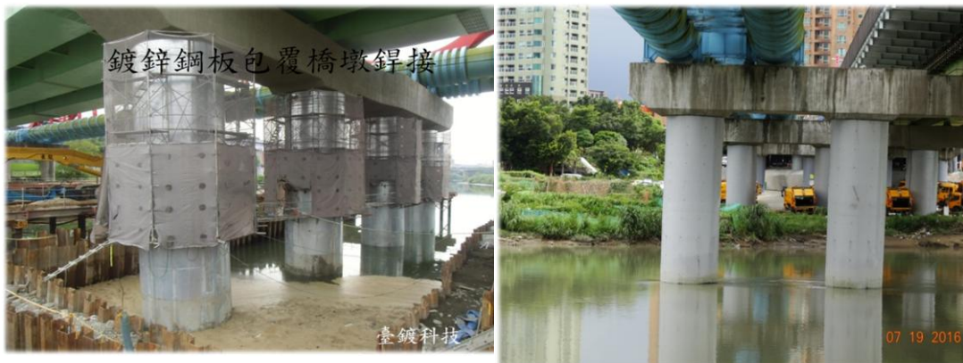
Figure 7. The piers of Yongfu water pipe bridge with steel jacket
