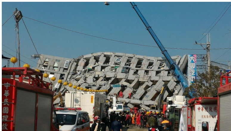
Fig.2 The collapsed 17-story Weiguan Jinlong residential building
