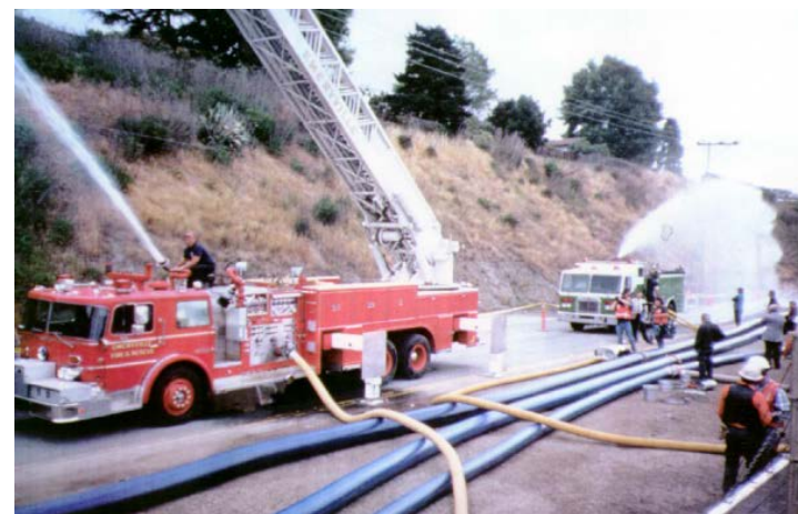
Temporary HDPE bypass lines for fault crossing (courtesy EBMUD)
