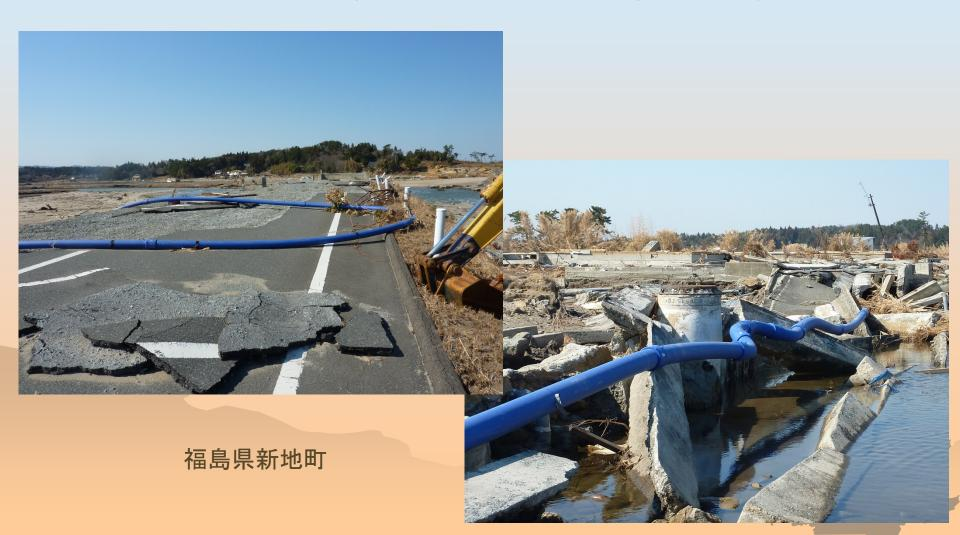
Deformation of pipeline by Tsunami (Bending angle at joint)
