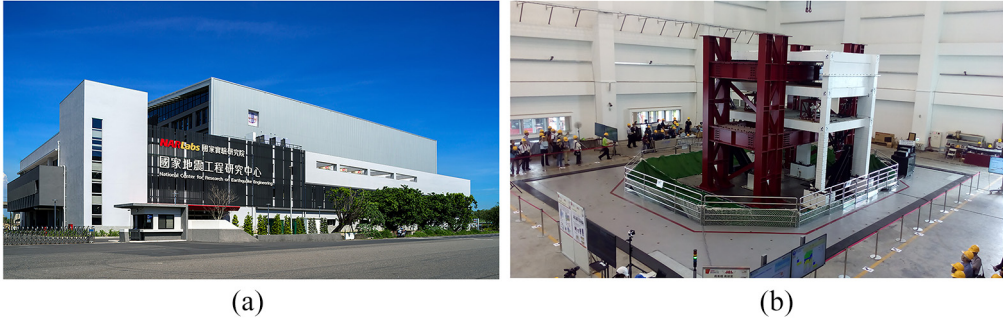
Figure 1. (a) NCREE Tainan lab and (b) The 8 m \times 8 m shaking table and the three-story RC building (the white part).
