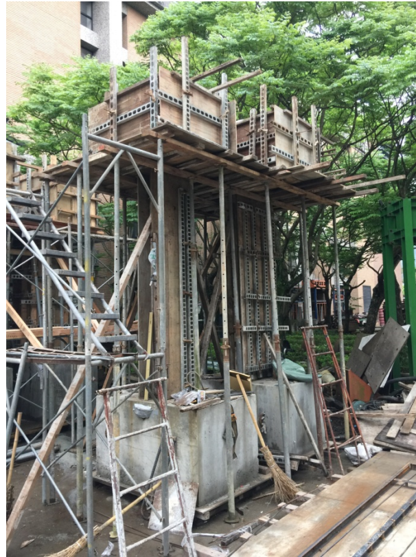
Formwork Assembly Completed
