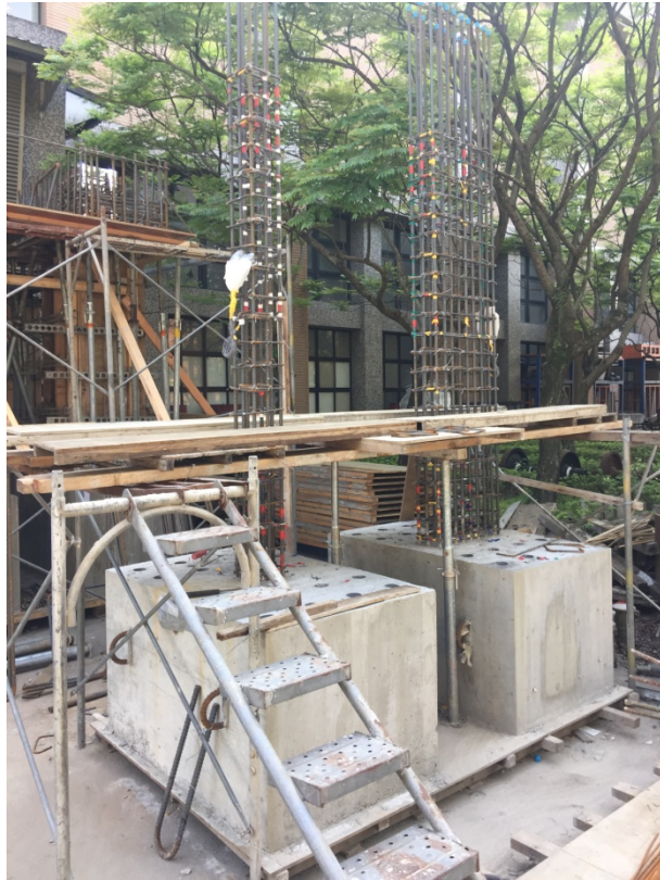
Rebar Installation Completed
