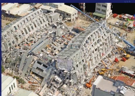
Collapse of Weiguan Jinlong Complex in the ML-6.6 Meinong Earthquake
