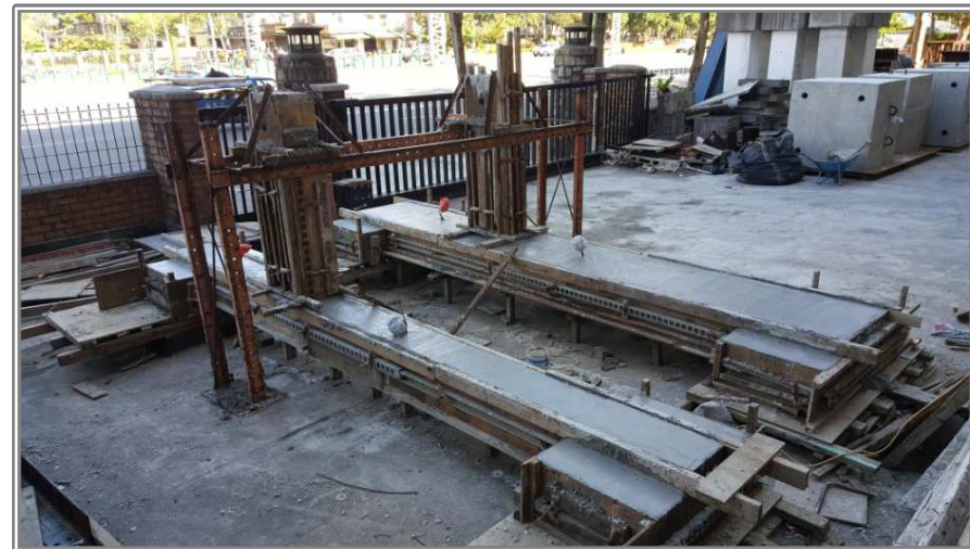
Concrete Pouring Completed
