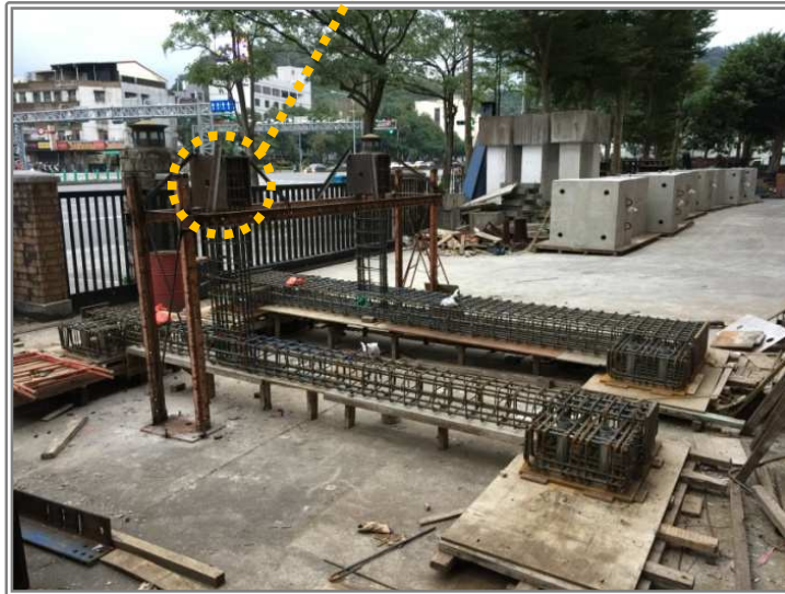
Rebar Installation Completed
