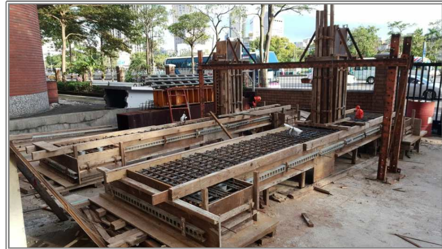
Formwork Assembly Completed
