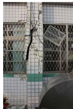
(a) 窗台柱剪力破壞
