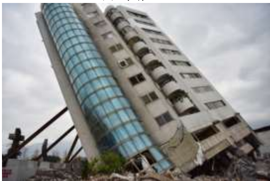
(c)建築倒塌傾斜
